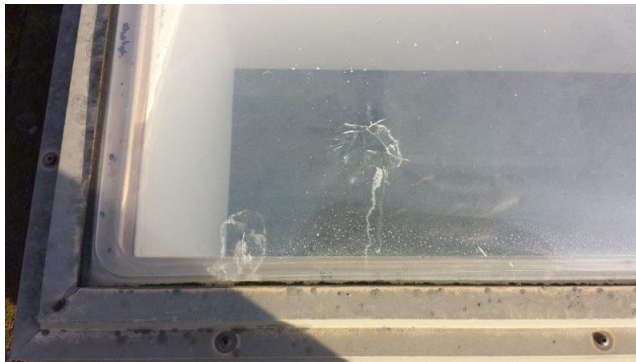
Roof 6 Damaged Skylight
