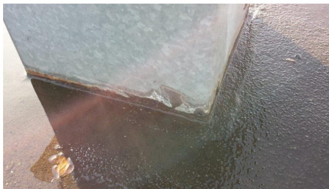
Roof 8 corrosion of sheet metal vent
