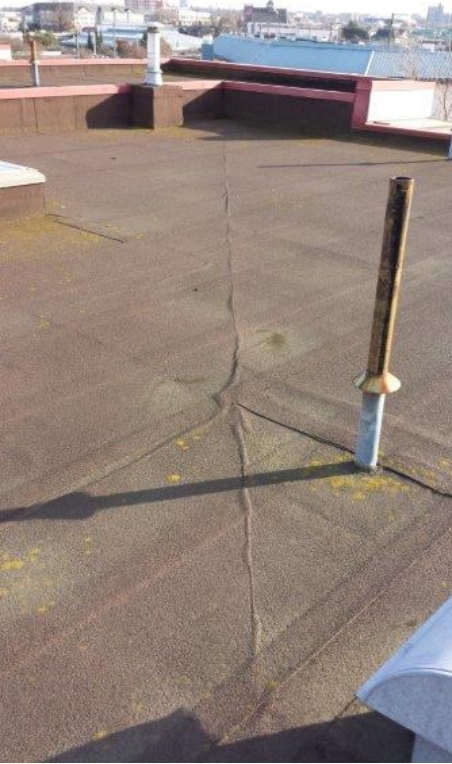
Roof 1 Wrinkled membrane
