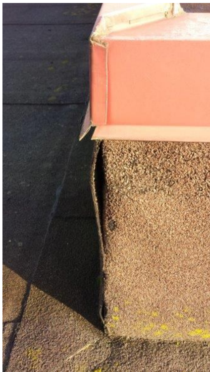
Roof 8 corrosion of sheet metal vent
