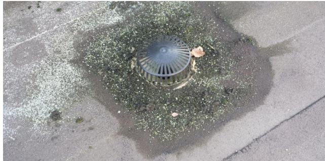
Roof 3 Debris around drain
