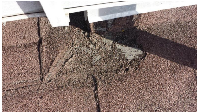
Roof 2 Missing granulars on membrane surface
