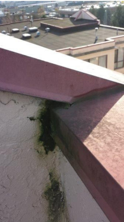
Roof 1 Wrinkled membrane
